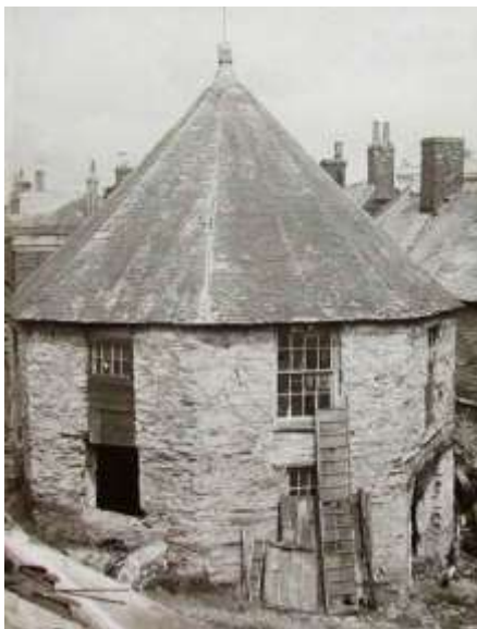
The Cockpit Chapel—Cornish Story
